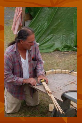
waagaadoowaatigoog(end pieces) aresteamed, bent,formed, and wrappedtight
